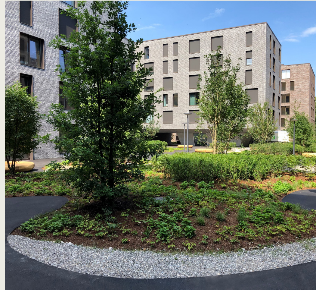
A real estate project of a Swiss insurer (2019): The greenhouse gas emissions from the building in operation are just under 1 kg CO 2 /m 2 (the target for new builds set by the Swiss Society of Engineers and Architects is 2.5 kg CO 2 /m 2 ).
